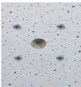
Fig. 14: Holes ready for mounting
