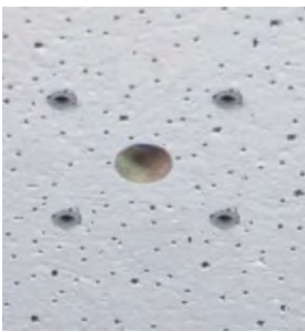
Fig. 16: Holes ready for mounting
